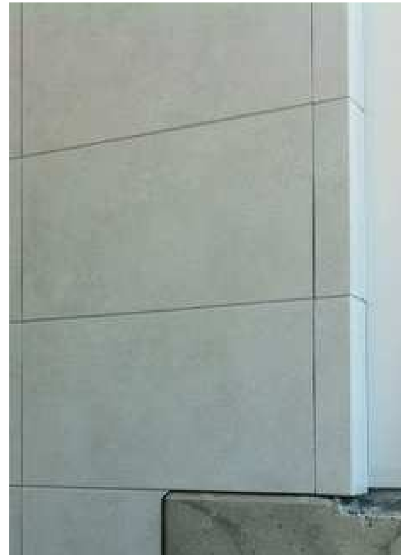
FIBER CEMENT BOARD - REVEAL PANEL SYSTEM
