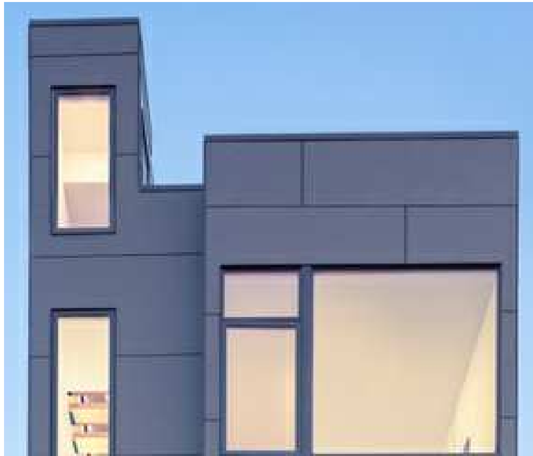
FIBER CEMENT BOARD - REVEAL PANEL SYSTEM
