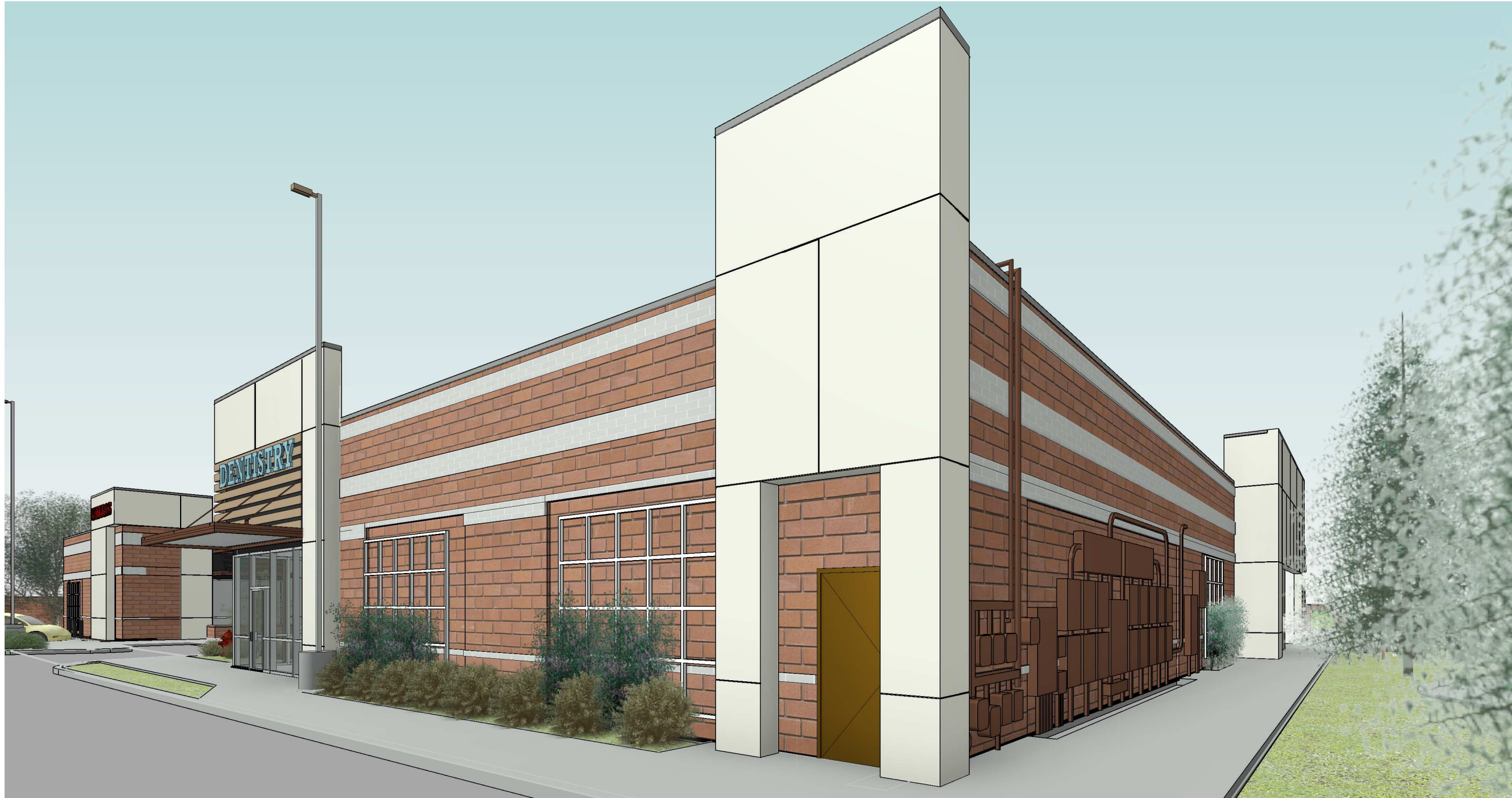
BUILDING 200 - VIEW FROM SOUTH
